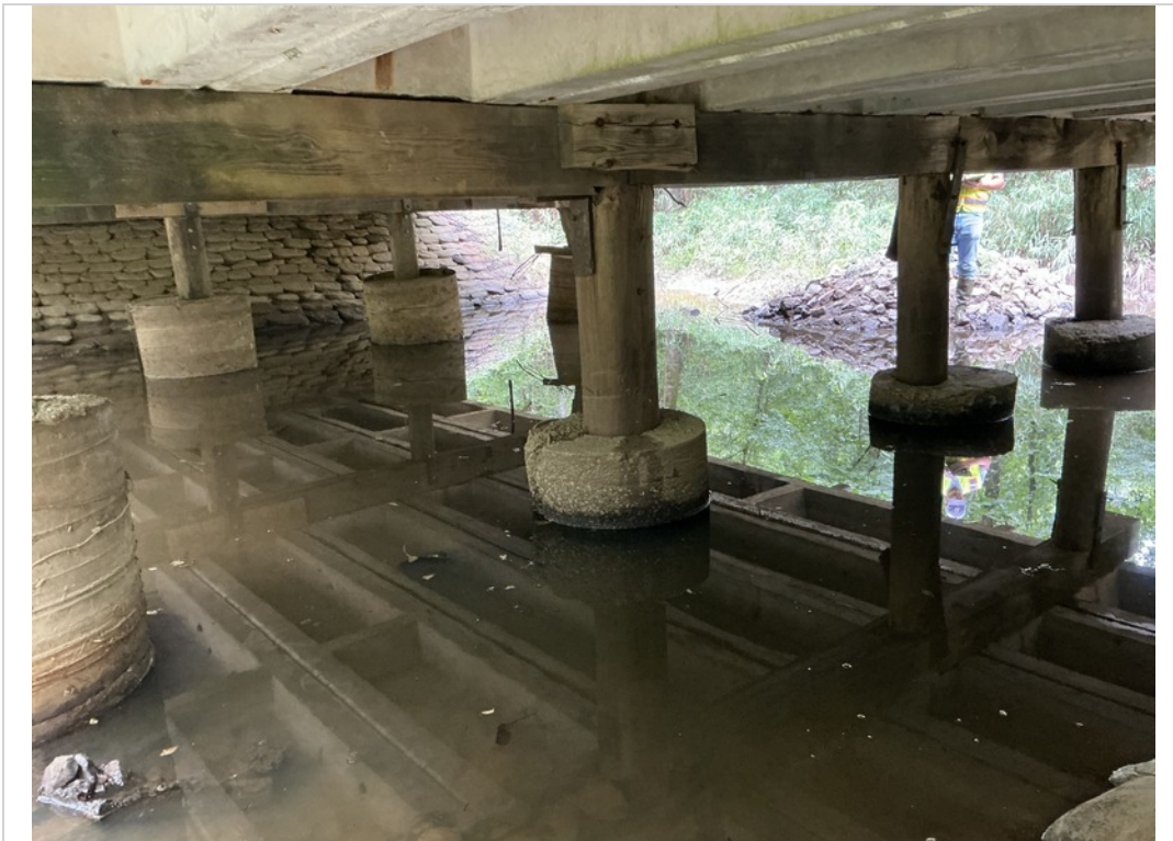
Bent 1 Looking Ahead
