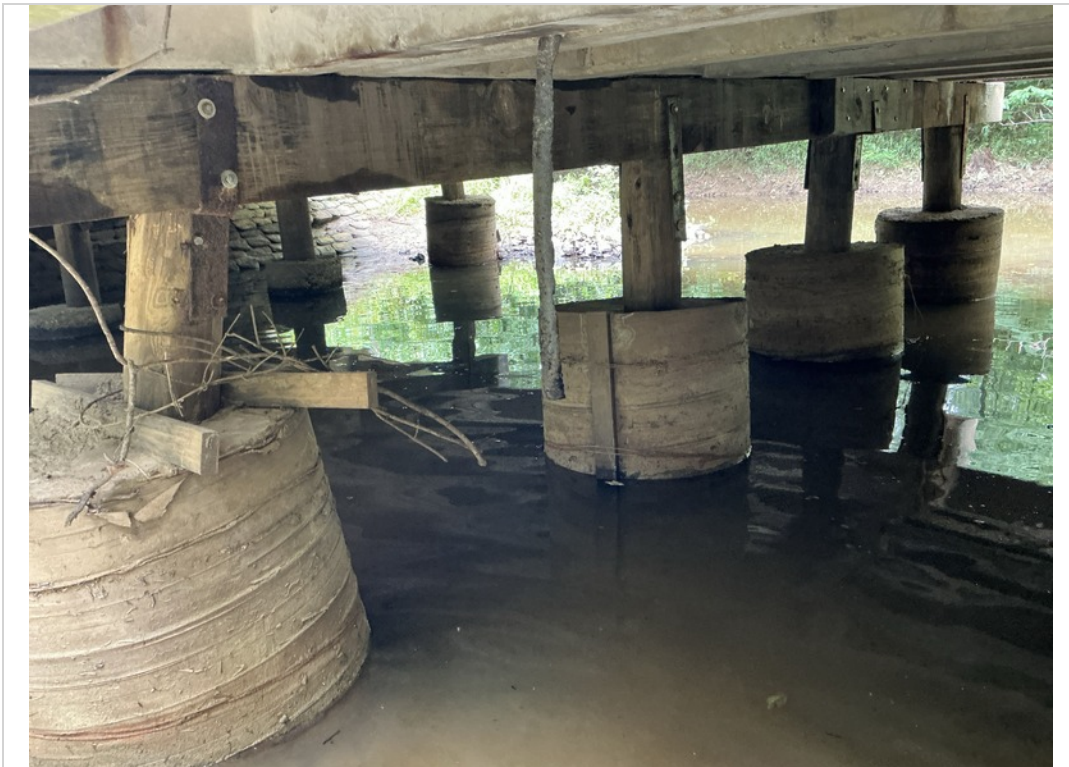
Bent 2 Replacement Looking Back Spliced Piles and New Cap
