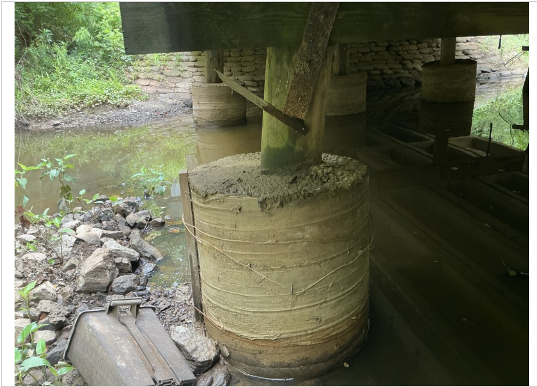
Bent 1 Pile A Replacement
